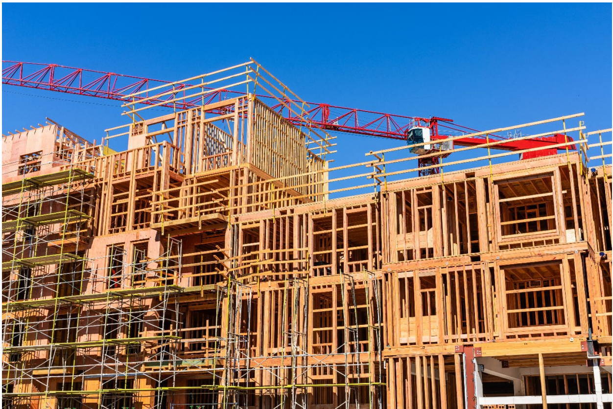
Noise generated from the construction of a housing development.
