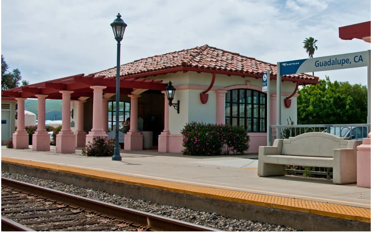
Guadalupe Amtrak Station (GUA). Credit: Amtrak.
