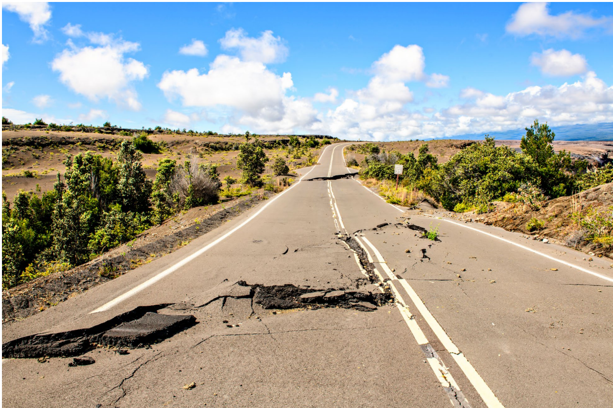
Earthquake causes major damage to roadway.
