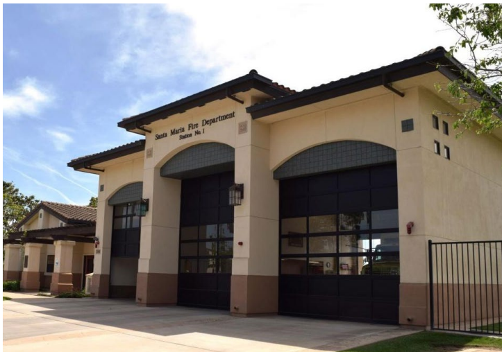
Santa Maria Fire Station No. 1
