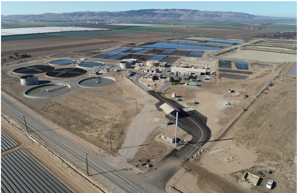
City of Santa Maria Wastewater Treatment Plant.
